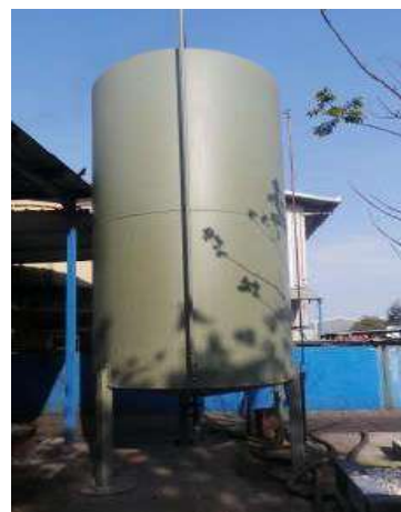
Gambar 6. Kondisi HSD Tank setelah di re-painting
